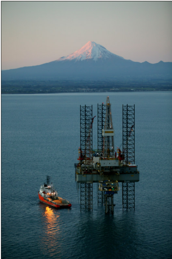
Figure 3 Installation and piling activities for the Pohokura Gas Platform were simulated using SDA for 8 individual years. The results were used to assess the impact of project slippage and to ensure the optimum use of the available weather windows.
